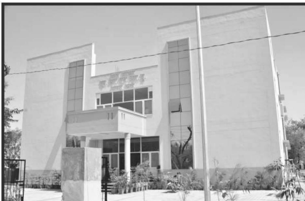
Building of Rajasthan MRHRU
