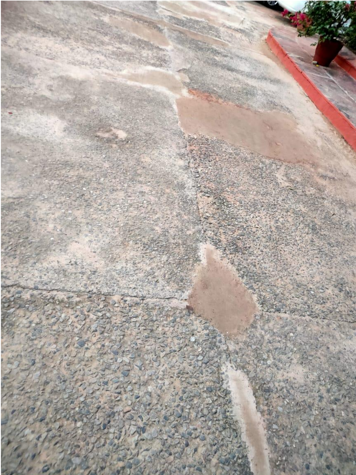
Potholes in the drive way filled during the cleanliness drive
