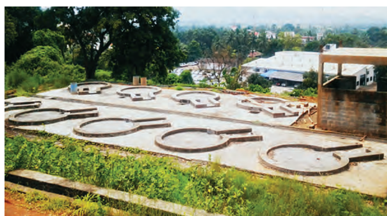
Corncrib No 2- Foundation work is completed
